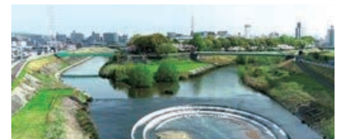
天白川と桶田川の合流点にある護床工 Construction designed for bed protection at the confluence of the Tempaku River and the Ueda River.
